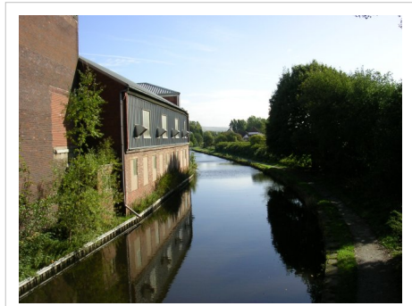
The Ashton Canal through Droylsden
